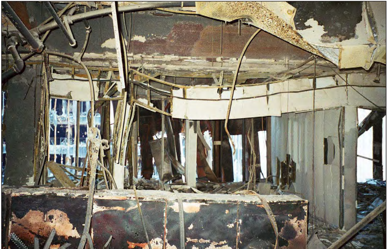
Figure 7-5 Interior damage at floor 20 of WFC 3.
