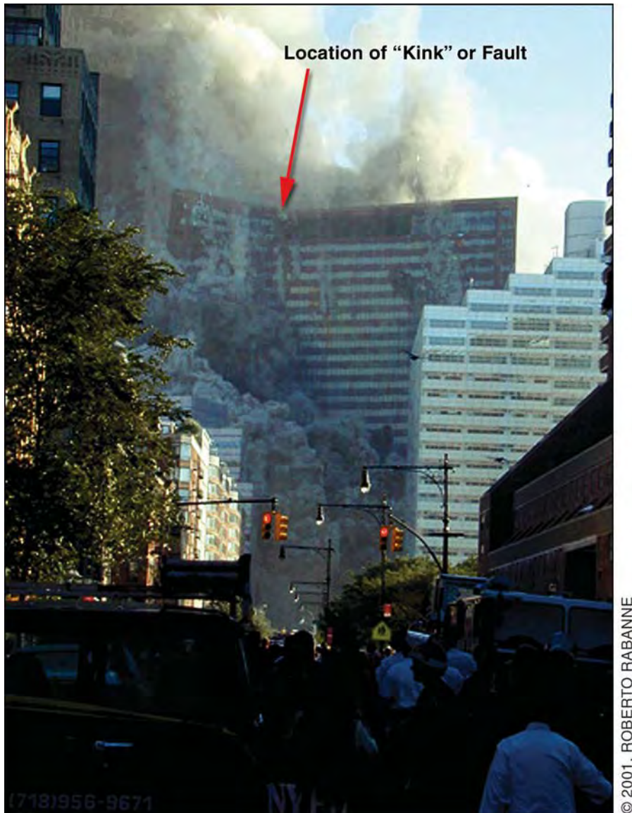
Figure 5-23 View from the north of the “kink” or fault developing in WTC 7.
