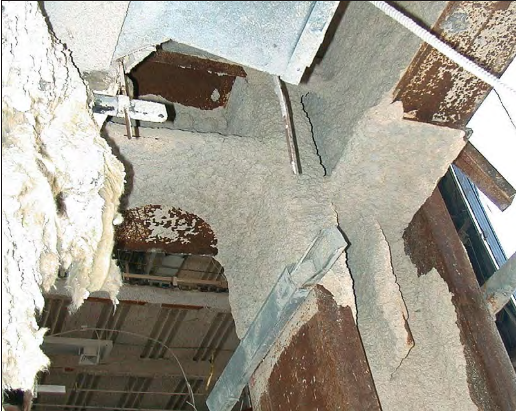
Figure 6-6 Moment-connected beams to columns.
