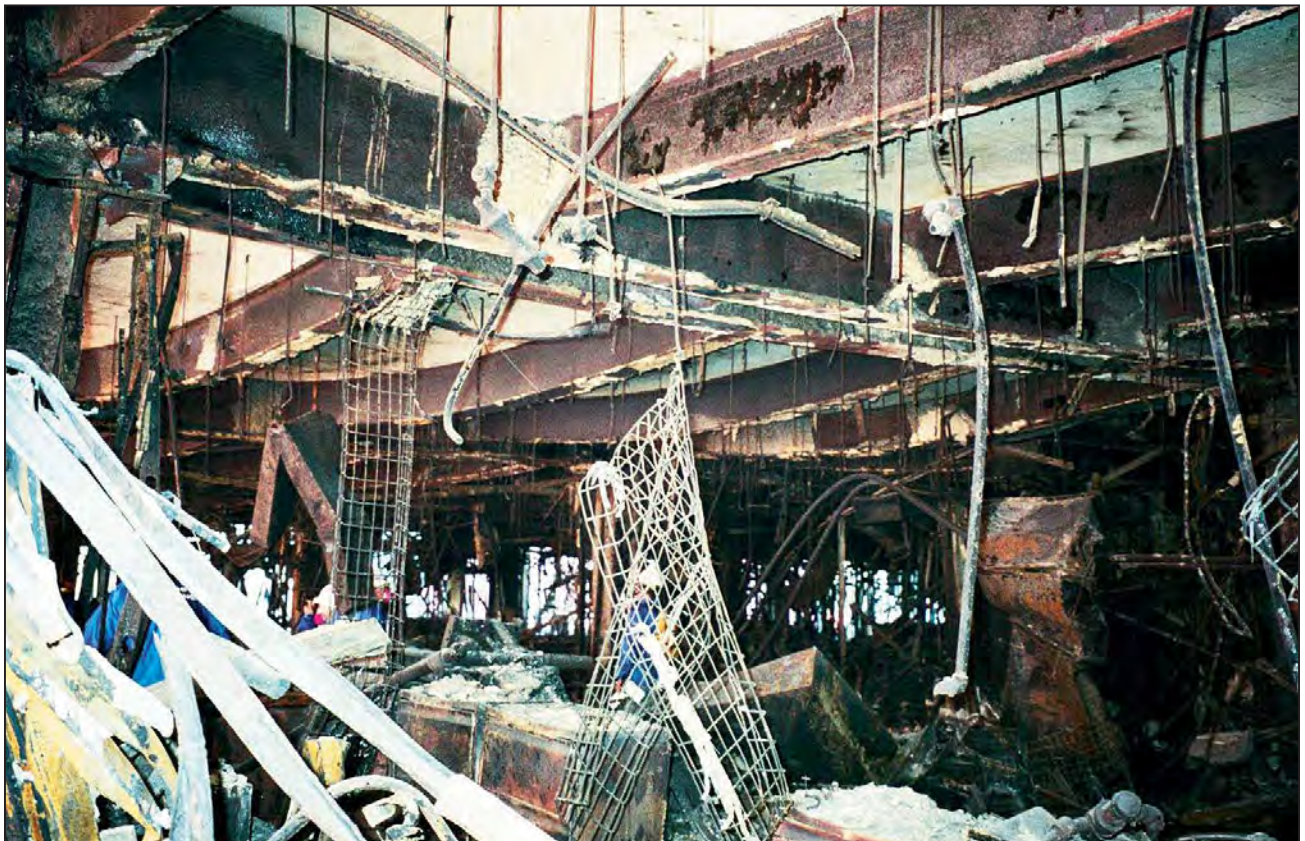
Figure 4-14 Deformed beams in WTC 5.
