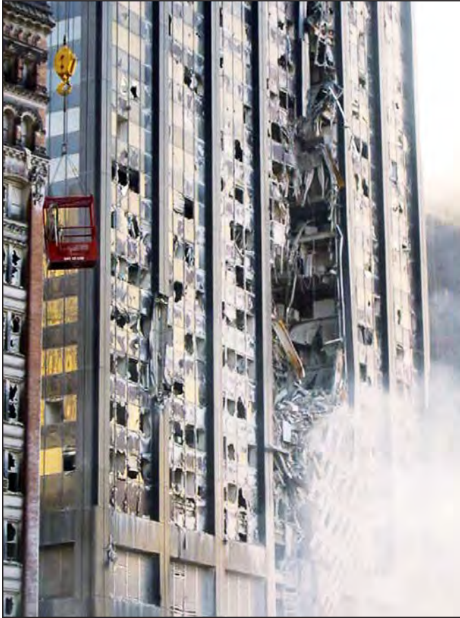
Figure 6-2 Closeup of area of partial collapse. Note debris accumulated at the bottom of the damage area, resting on the 8th floor. Area of initial impact is not shown in this photo.
