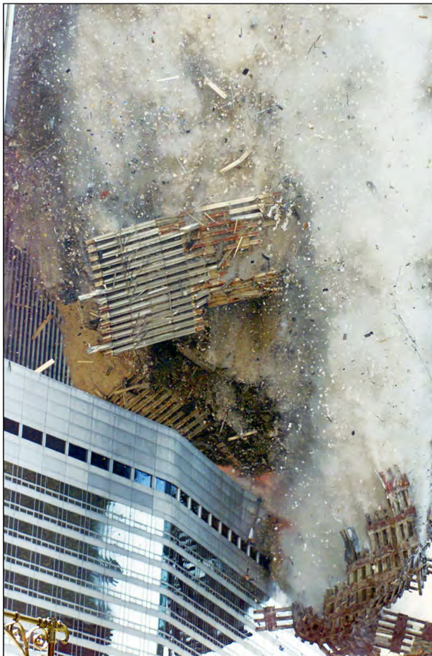
Figure 3-6 Exterior columns from the collapse of WTC 2 falling on the southern part of WTC 3.
