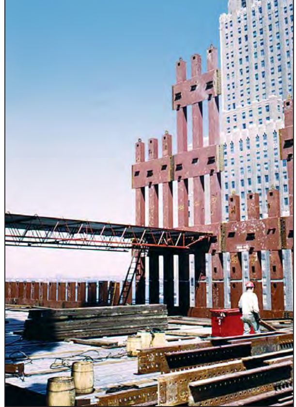
Figure 2-8 Erection of floor framing during original construction.
