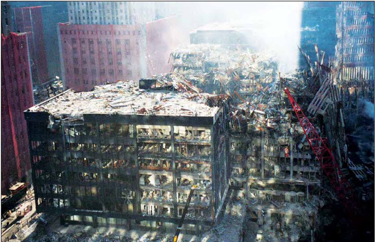
Figure 4-9 Impact damage to WTC 6.
