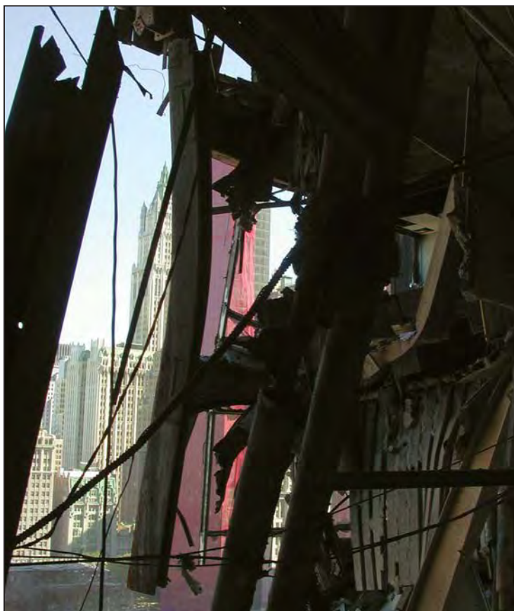
Figure 6-9 Suspended column D-8 at the 15th floor. Note separation at column splices.
