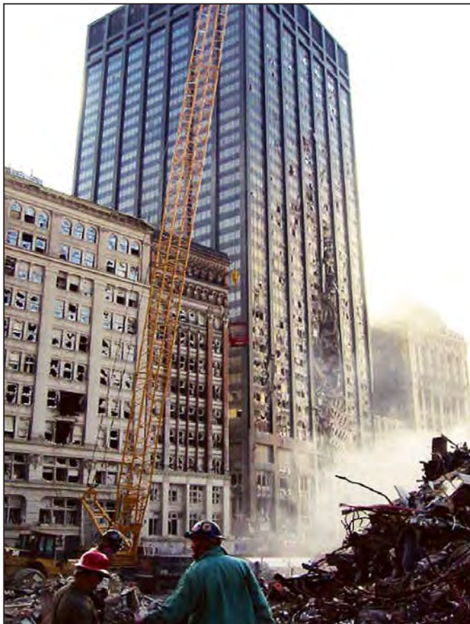
Figure 6-1 North face of Bankers Trust building with impact damage between floors 8 and 23.
