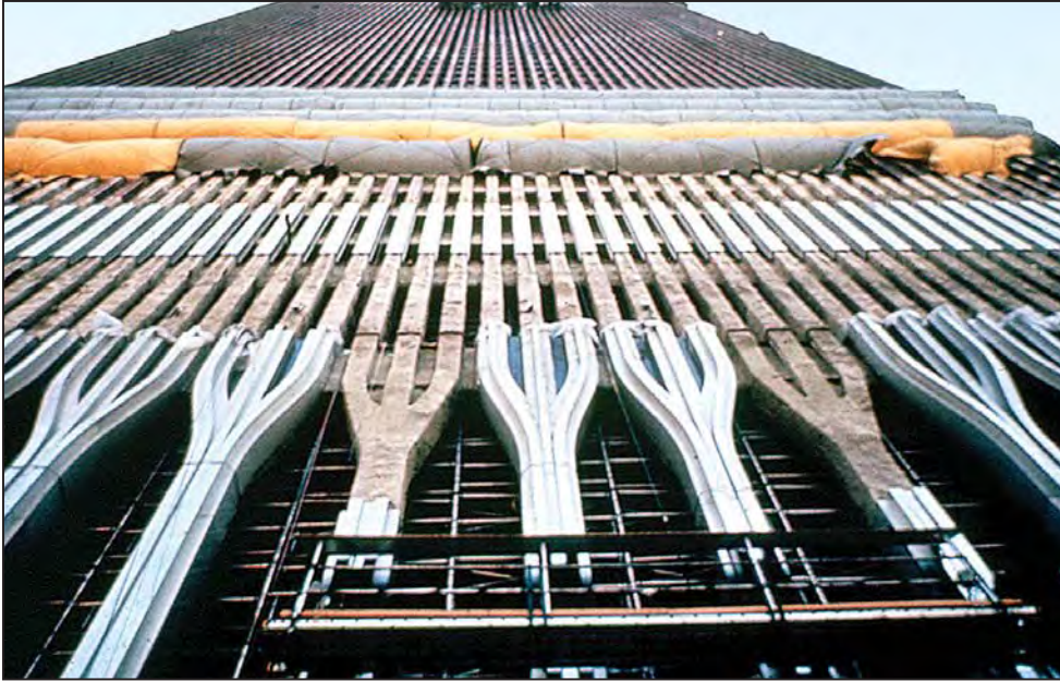
Figure 2-4 Base of exterior wall frame.
