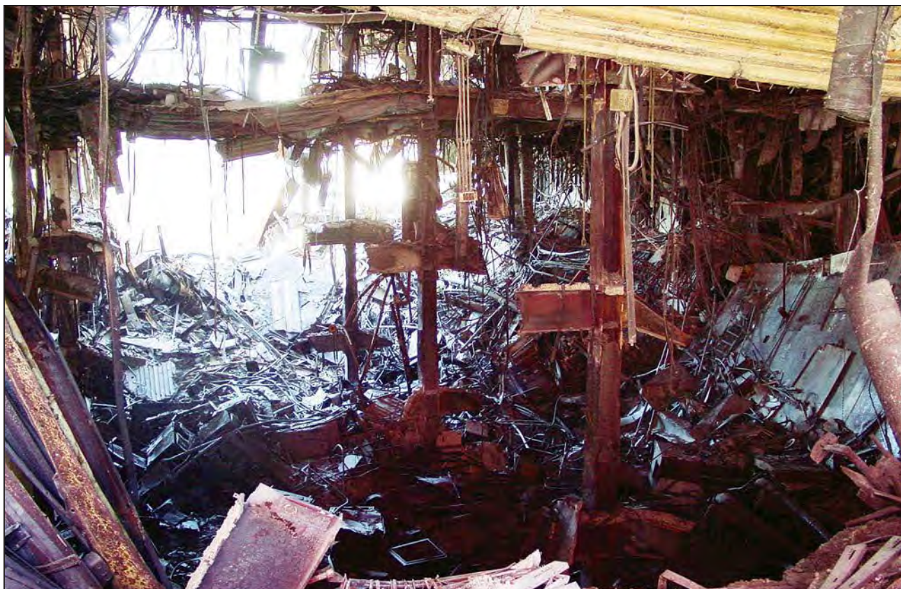
Figure 4-20 Internal collapsed area in WTC 5.
