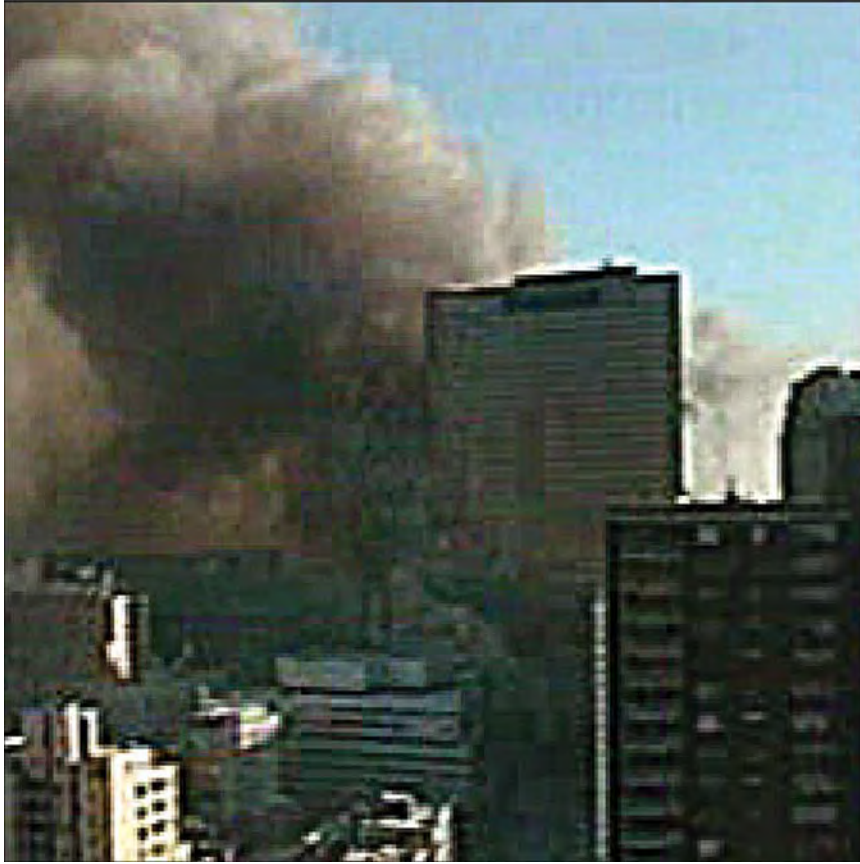
Figure 5-21 East mechanical penthouse collapsed. (From video.)
