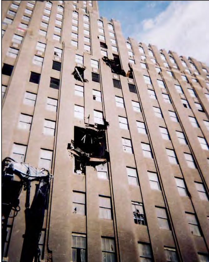
Figure 7-10 Verizon building – damage to south elevation (Vesey Street).
