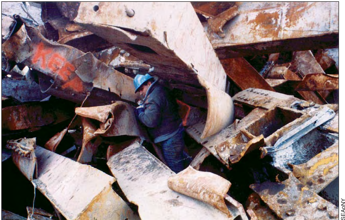
Figure D-4 Engineer climbing in unprocessed steel pile to inspect and mark promising pieces.
