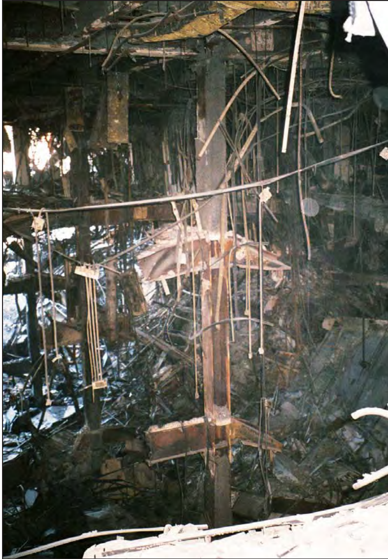
Figure 4-19 Internal collapsed area in WTC 5.
