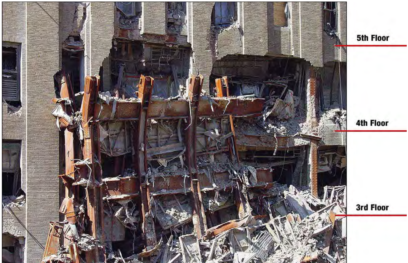
Figure 7-7 Verizon building – damage to east elevation (Washington Street) due to WTC 7 framing leaning against the building.
