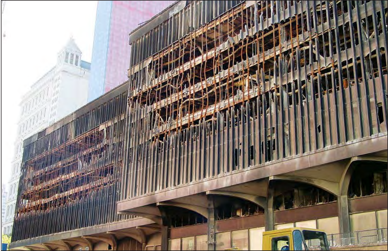
Figure 4-11 WTC 5 façade damage.
