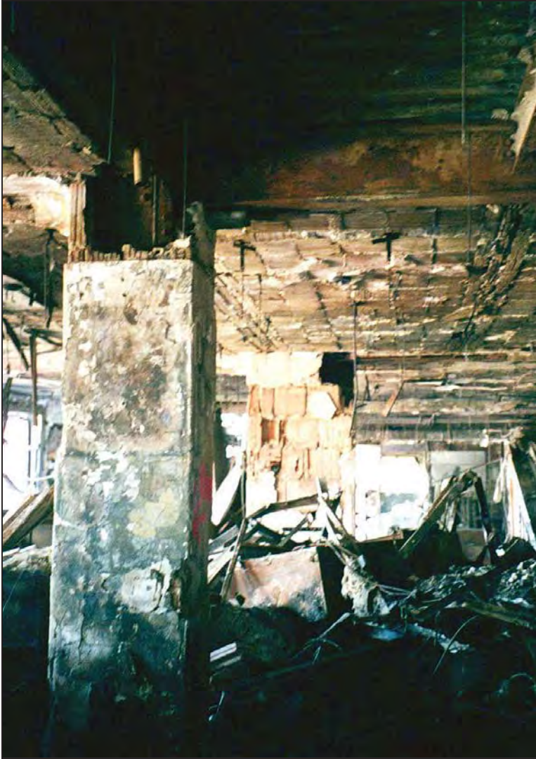
Figure 7-16 Buckling damage at top of column on floor 8 of 90 West Street. Note the loss of fire protection at the top of the column.
